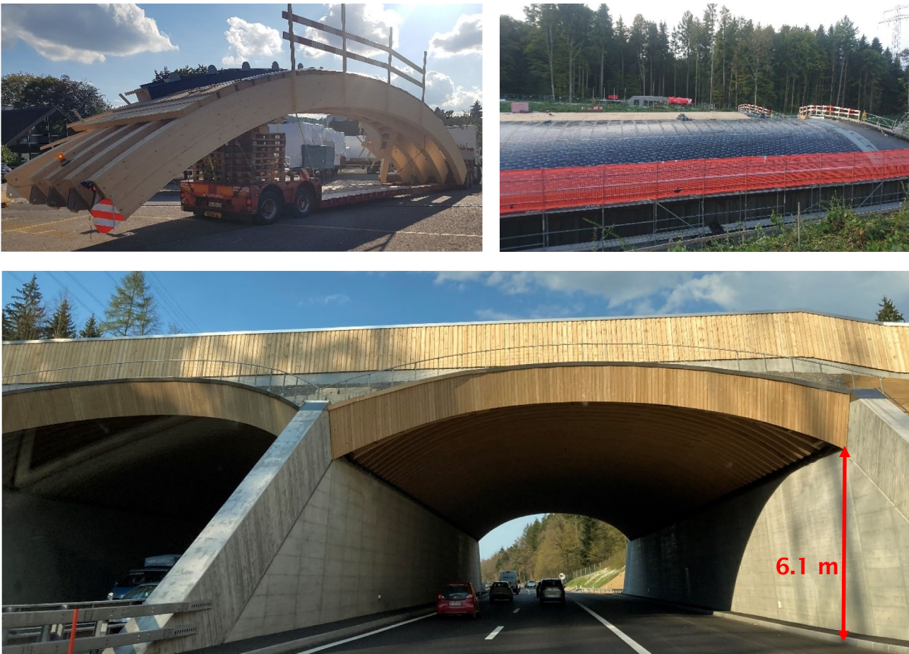
Fig. 1 An element of the wooden wildlife bridge on its way to the installation site (top left), the finished construction with the bitumen layer before filling the roof with earth (top right), and finally the frontal view of the entry (bottom)
