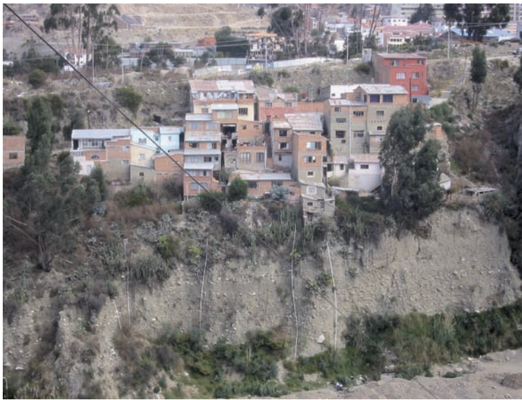
Figure 6: In La Paz, Bolivia, settlements have been built in areas highly exposed to landslides. (Photo by Annika Salmi)
