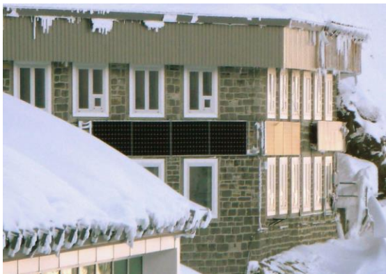
Figure 2a: Jungfrauoch research building with existing PV-installation (from 1993) on the right façade and new (2014) PV modules on the left façade.
