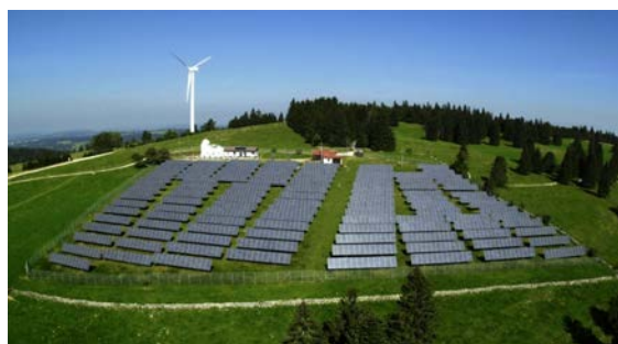
Figure 1: PV plant Mont-Soleil
