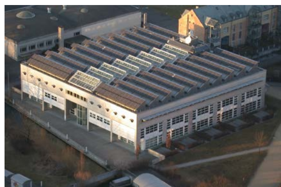
Figure 3: Roof-top PV plant in Burgdorf consisting of three areas: Building East (right), Building west (left) and
