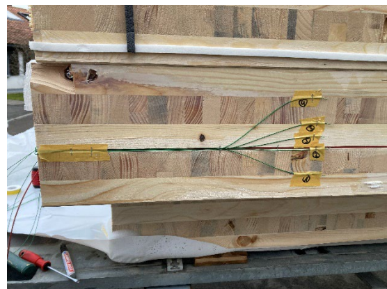
Figure 12: temperature sensors onsite
