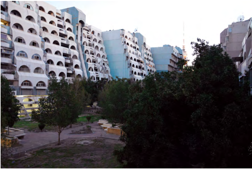
Figure 7: Al-Sawaber, Kuwait City. Photograph taken by Laura Hindelang before demolition
