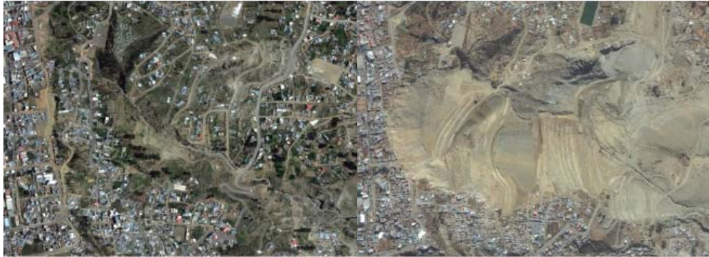
Figure 4: The 26 February 2011 megadeslizamiento, a big landslide that devastated large parts of the city of La Paz. Left: the area before the catastrophe; right: the area afterwards. (Photos courtesy of Gobierno Autonomo Municipal de La Paz [GAMLPA])
