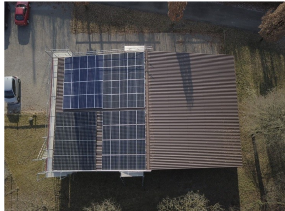
Figure 2a: Four PV technologies were installed.
